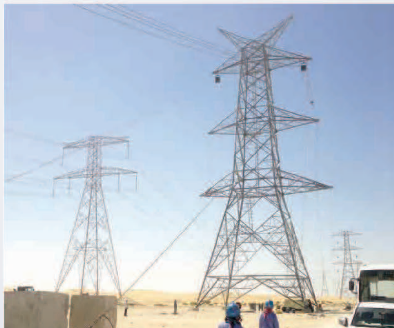
Stringing work in Dubai Consultancy project
