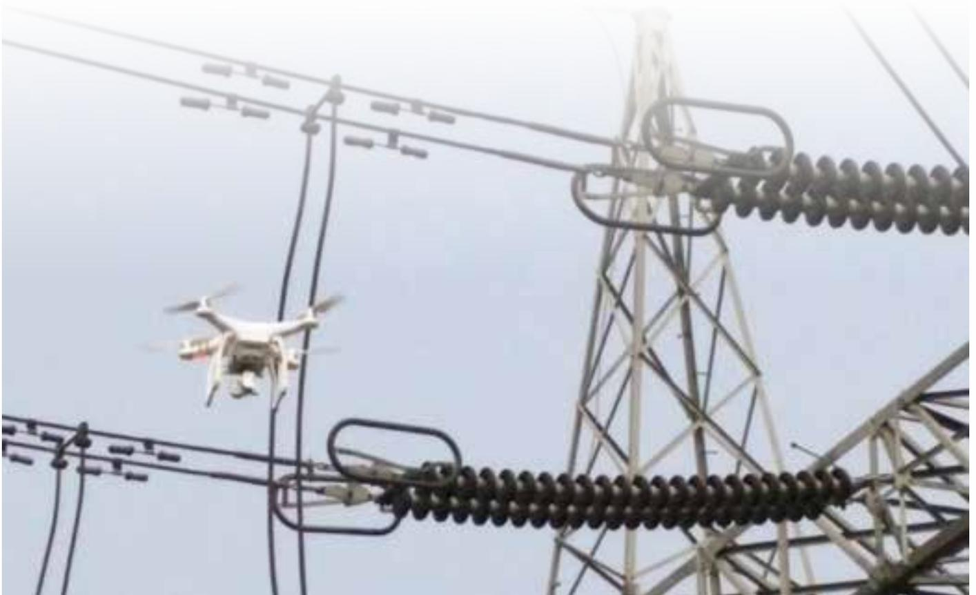
*Surveillance of Transmission Assesst by Drone*
