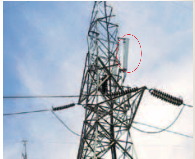
Telecom antenna on transmission tower
