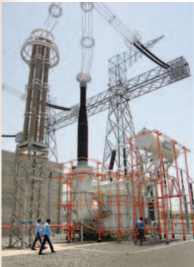
1200kV transformer
