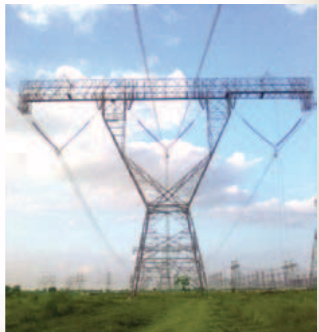
1200 kV Transmission Tower
