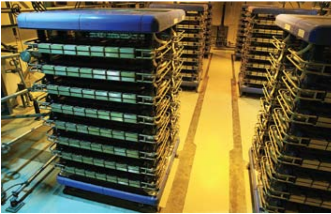
HVDC Valve Hall
