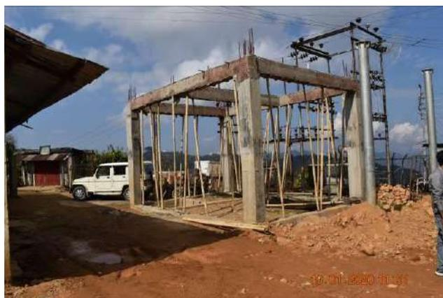
Refilling and leveling work at new 33/11 kV Substation at Longleng Town
