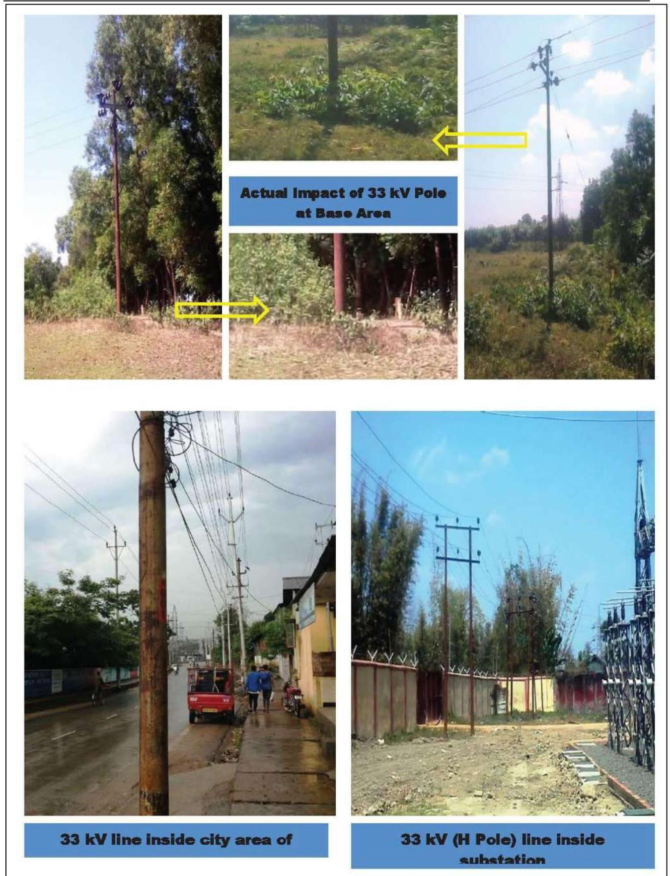
Figure 4.8: 33 kV Lines (Single & H Pole) Depicting Base Area Impact
