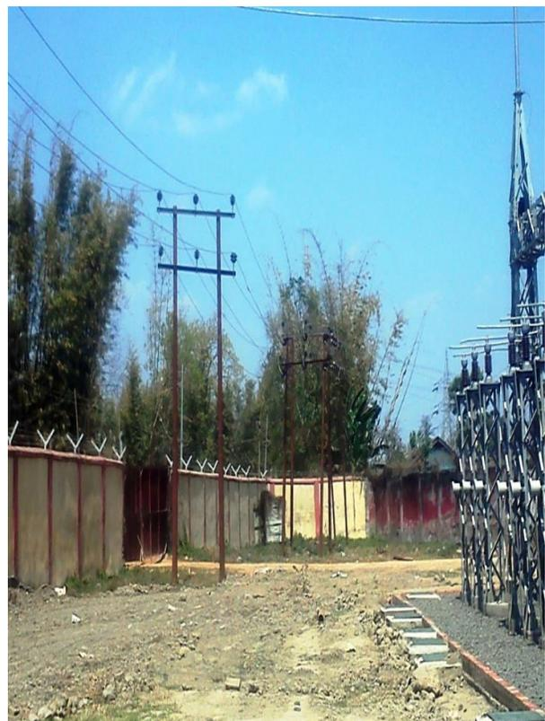
**33 kV (H Pole) line inside substation**
