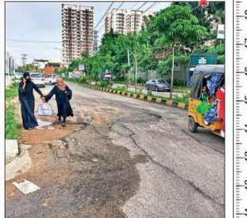
Near Essen Presidential building, Kokapet, four and two wheelers are taking blind turn on the wrong side of the road which is a one-way. This creates a risky situation for vehicles coming in and for pedestrians walking down the road. Adding to this, potholes and open manholes could lead to a fatal accident. — Mithlesh Kumar
