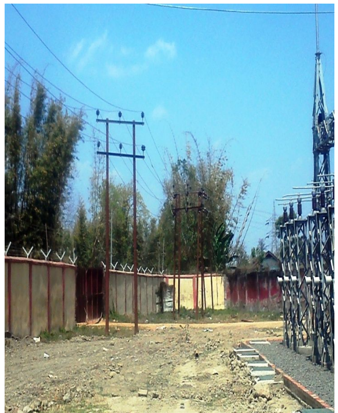
33 kV (H Pole) line inside substation
