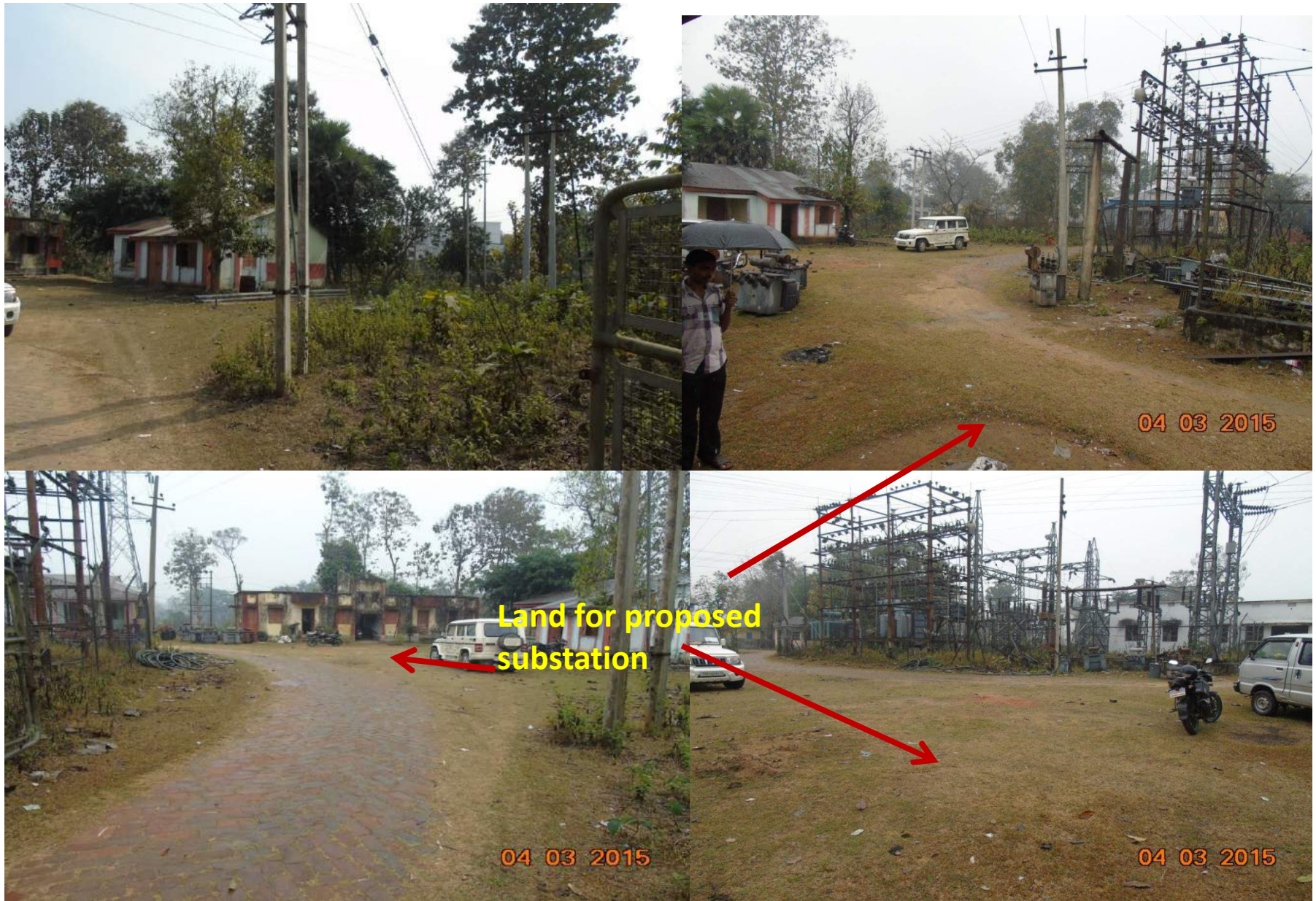
VIEW OF SATCHAND 66 KV EXISTING SUBSTATION
