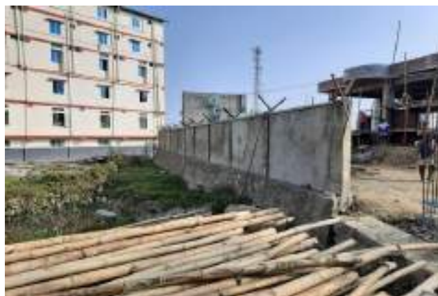
Retaining Wall at 33/11 kV Pishum (GIS) S/s
