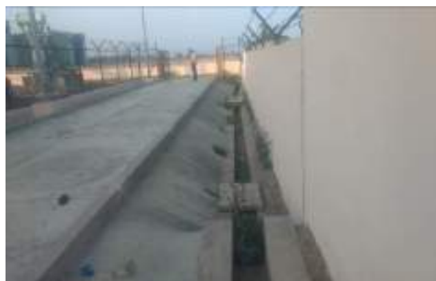
Drainage and Sewage system within the 33/11 kV Hiyanthang Substation
