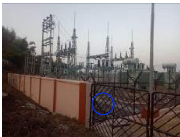
Stone Pitching at 33/11 kV Leimapokpam S/s
