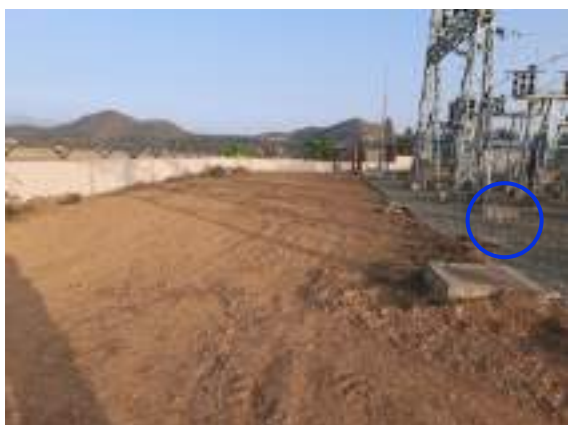
Stone Pitching at 33/11 kV Hiyanthang S/s
