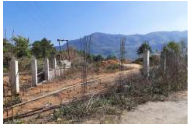
Boundary Walls at 132/33 kV Gamphajol Substation
