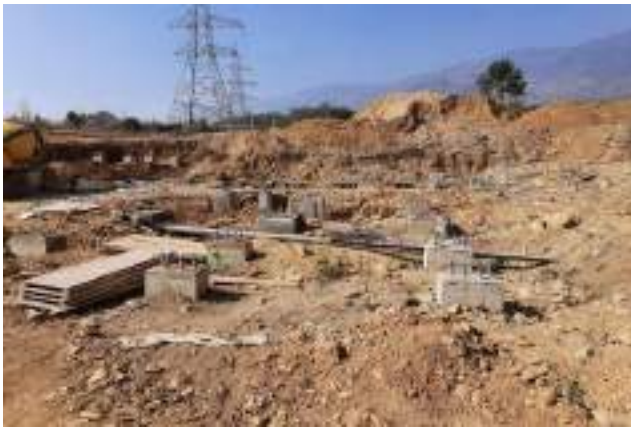
Earth cutting and Surface levelling at 132/33 kV Gamphajol Substation
