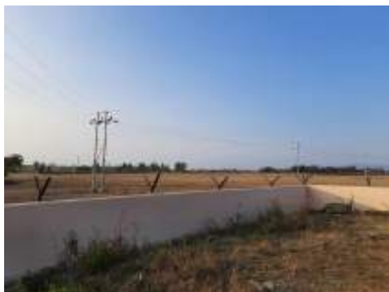
RRM Wall at 33/11 kV Hiyanthang S/s
