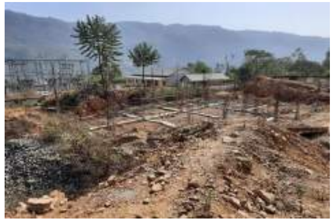
Earth cutting and Surface levelling at 132/33 kV Gamphajol Substation
