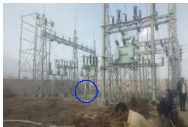
Stone Pitching at 33/11 kV Kwatka S/s
