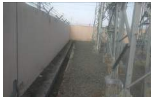
Drainage within the 33/11 kV Kwakta Substations
