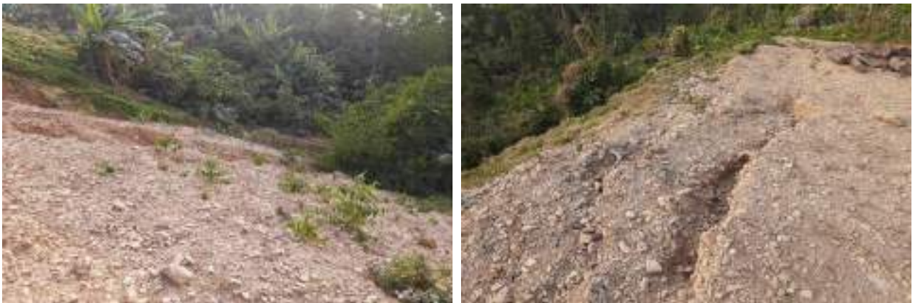
Landslips due to soil erosion
