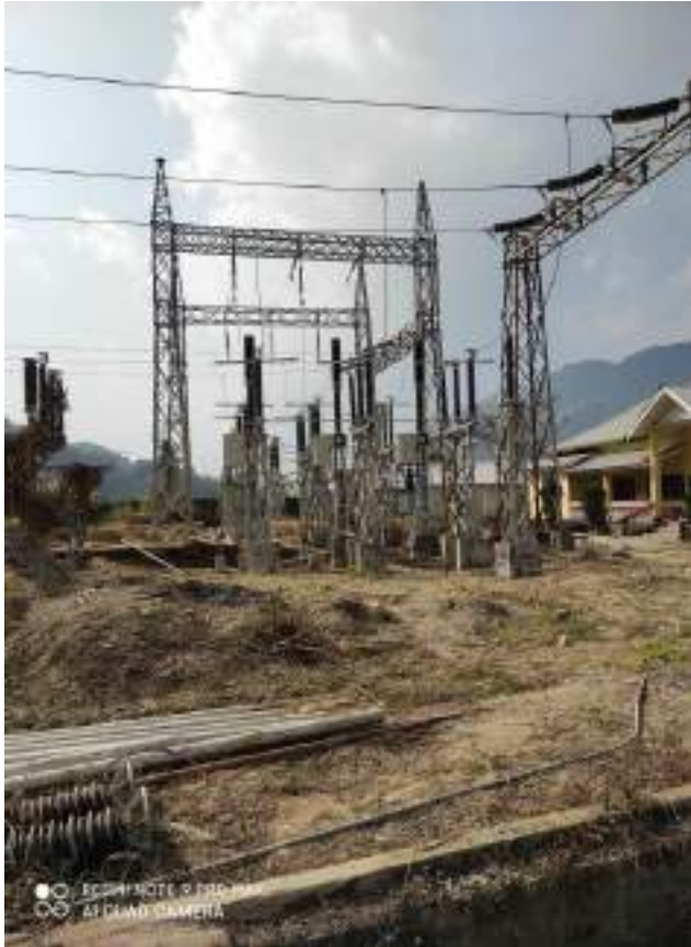
Existing 132/33 kV Substation at Rengpang (Bay Extension)
