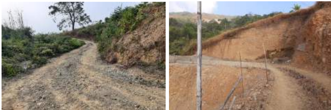
Proposed Approach road at 132/33 kV Tamenglong Substation
