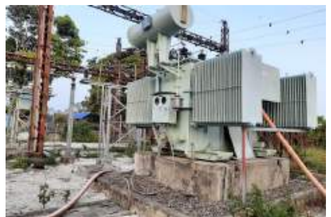
Existing 32/11 kV Substation at Leimakhong (Augmentation)
