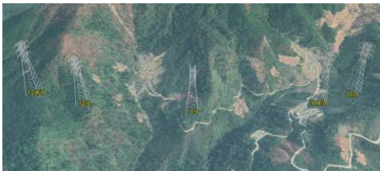
Increase in Length of Span to minimize tree cutting in Valley Area
