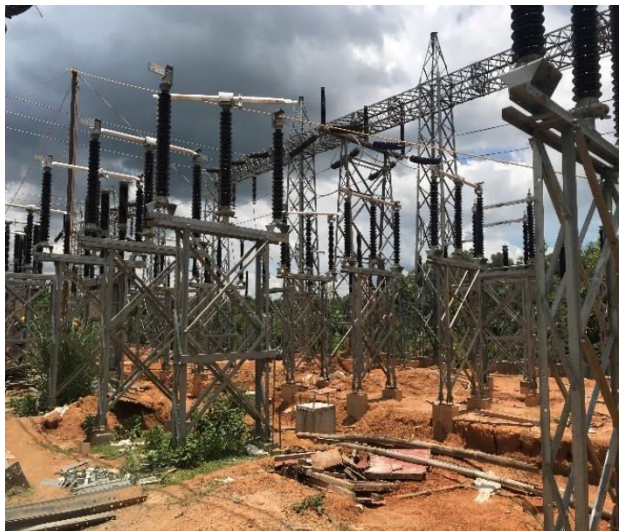
132/33 kV Belonia S/S – Equipment Erection
