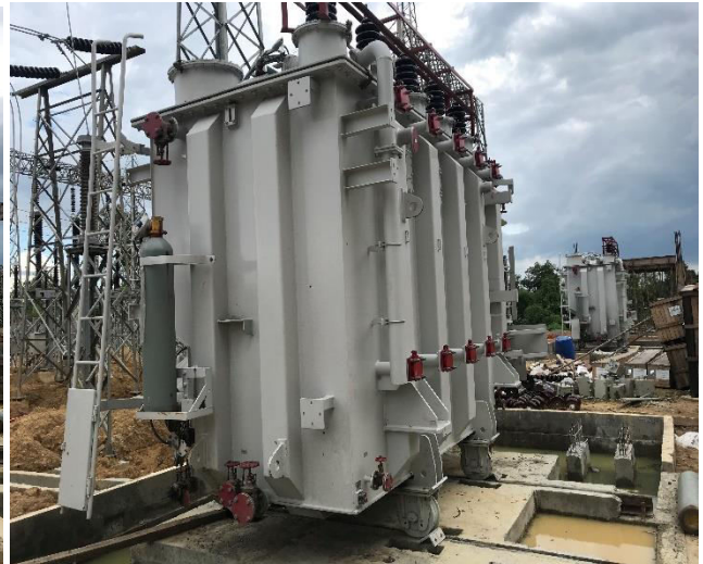
Transformer Erection with Oil Pit at 132/33 kV Satchand S/S
