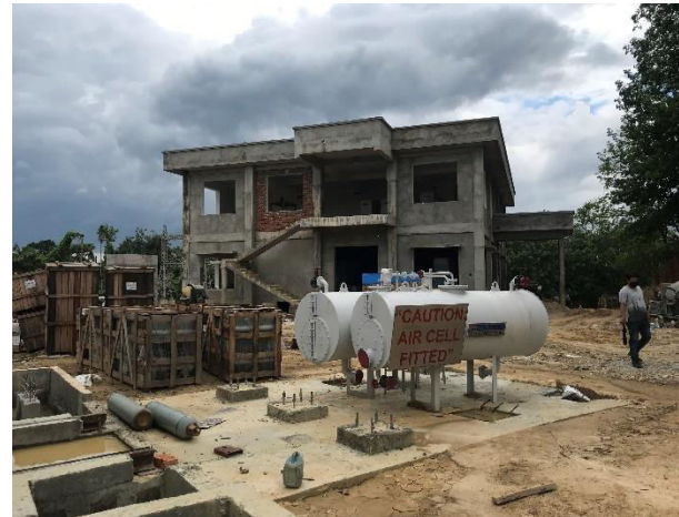
Air Cell Installed at 132/33 kV Satchand S/S
