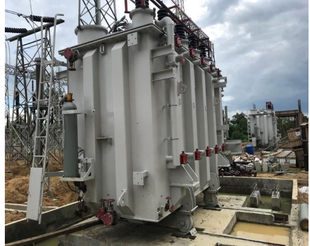
132/33 kV Satchand S/S – Control Room Building (Left) and Transformer Erection (Right)
