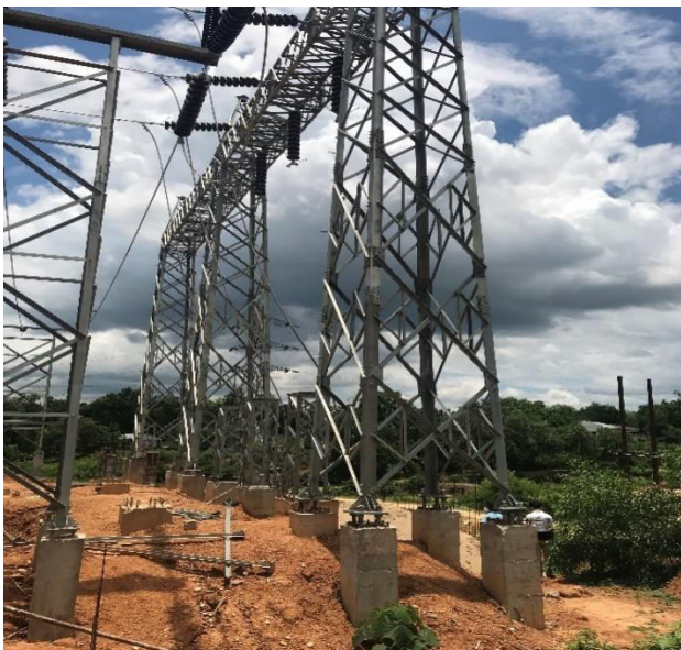
132/33 kV Belonia S/S – Equipment Erection
