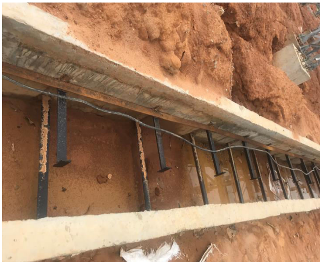
Trench Construction (Left) and Transformer Foundation with Fire Wall (Right) at 132 kV Bagafa S/S
