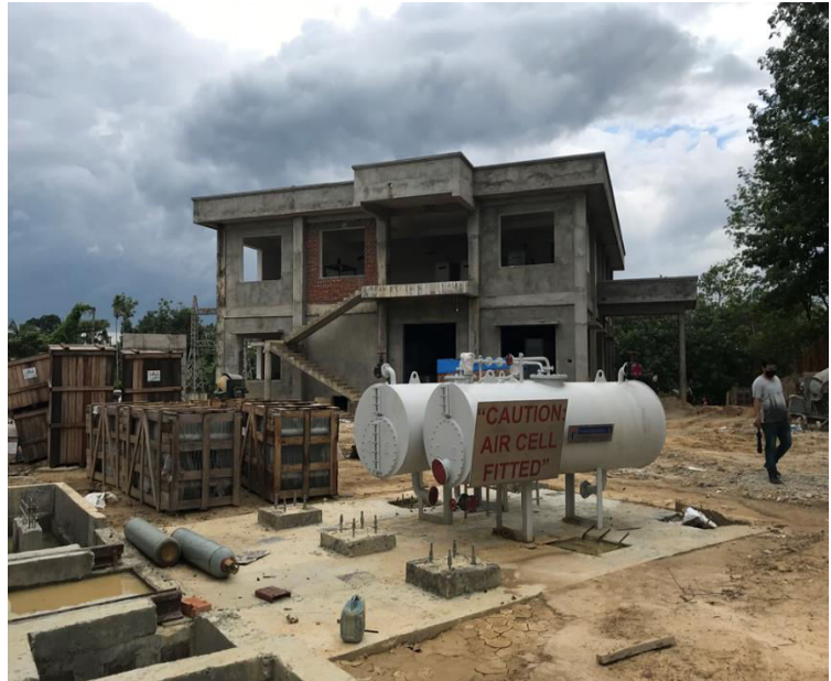
1132/33 kV Satchand S/S – Trench Construction (Left) and Air Cell for Transformer (Right)
