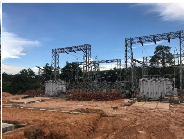
Transformer Erection with Oil Pit at 132/33 kV Sabroom S/S
