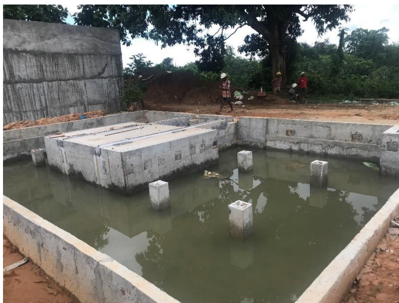
Transformer Foundation with Fire Wall at 132 kV Bagafa S/S
