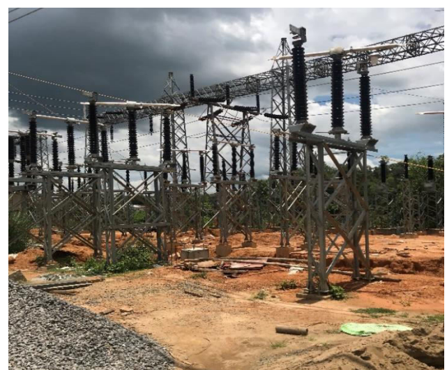
132/33 kV Belonia S/S – Equipment Erection
