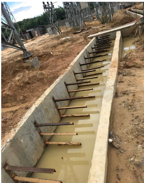
1132/33 kV Satchand S/S – Trench Construction (Left) and Air Cell for Transformer (Right)
