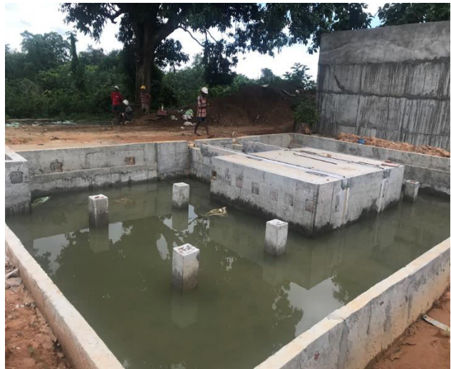
Trench Construction (Left) and Transformer Foundation with Fire Wall (Right) at 132 kV Bagafa S/S
