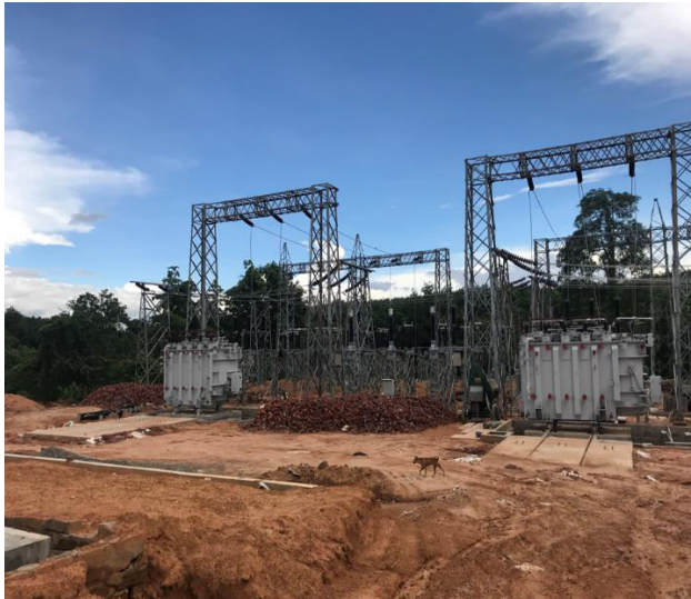
132/33 kV Sabroom S/S Transformer Erection (Left) and Drainage System (Right)
