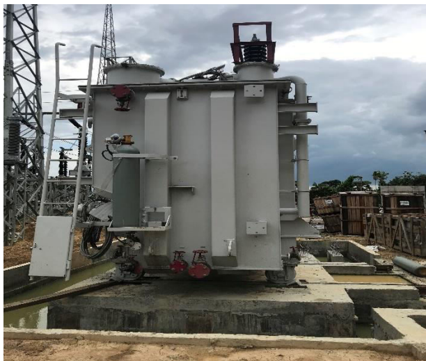
Transformer Erection with Oil Pit at 132/33 kV Satchand S/S
