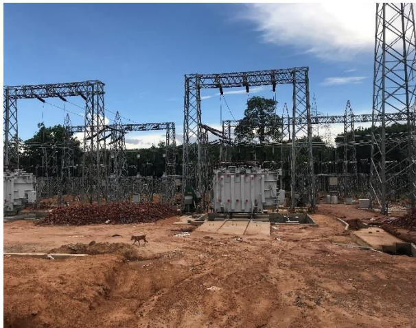
Transformer Erection with Oil Pit at 132/33 kV Sabroom S/S
