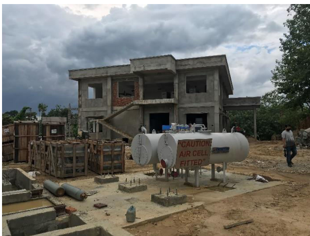
Air Cell Installed at 132/33 kV Satchand S/S
