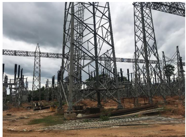
132/33 kV Bagafa S/S – Equipment Erection (Left) and Tower Erection (Right)
