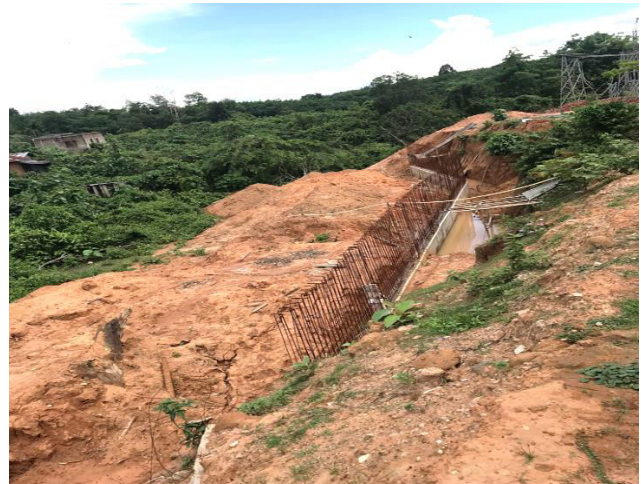
132/33 kV Sabroom S/S Building (left) and Retention Wall Construction (Right)
