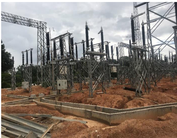
132/33 kV Bagafa S/S – Equipment Erection (Left) and Tower Erection (Right)
