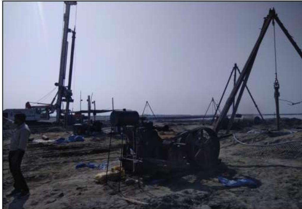
**Pile foundation work at Brahmaputra river for construction of 132 kV Rupai-Chapakhowa Electric Line**
