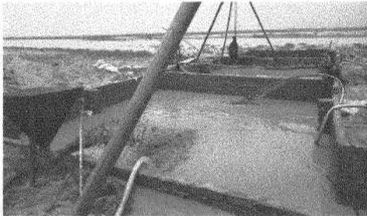
Fig: Bentonite Mixing Tank
