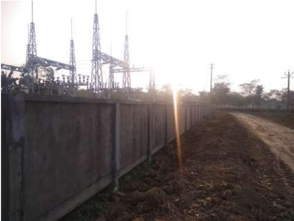
FIGURE 5-11 A PHOTOGRAPH SHOWING BOUNDARY WALL OF ROMAI SUBSTATION TO AVOID NUISANCE TO NEARBY PROPERTIES
