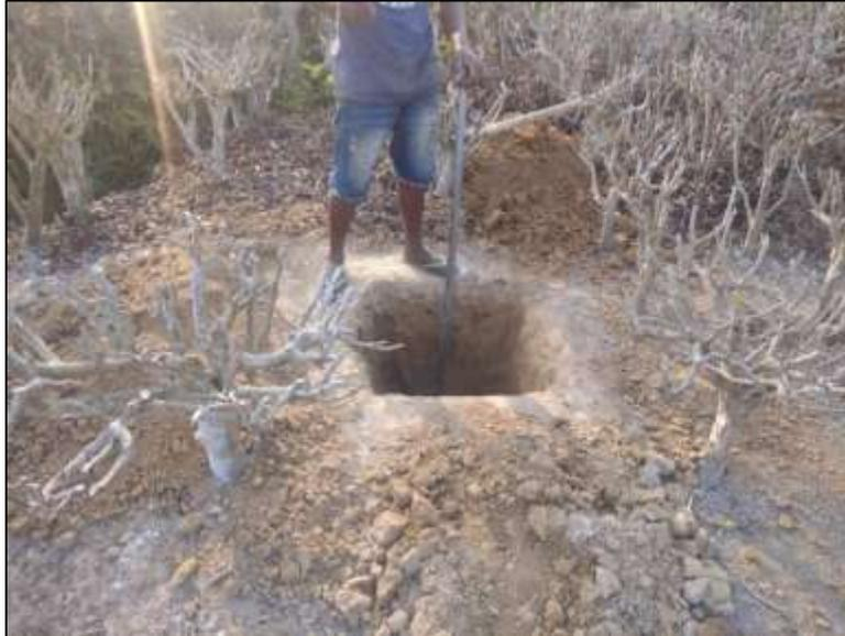
A photo showing excavation for construction of a pole for 33 kV Dibrugarh- Romai distribution line
