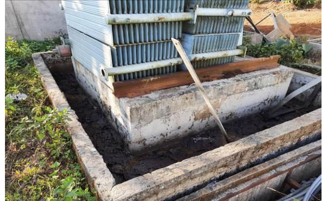
Oil Spill Containment Systems at 33/11 kV Lumshnong and Latyrke S/S
