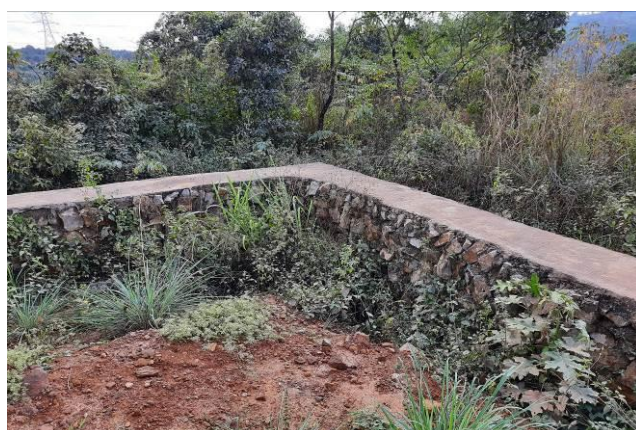
Retaining Wall at Tower AP-42A/0
