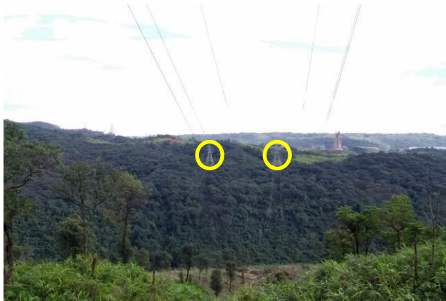
Tower on Hill Top to Minimize Tree Cutting
