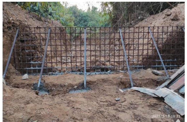
Nala Cleaning and Grating Work Carried out by PGCIL
