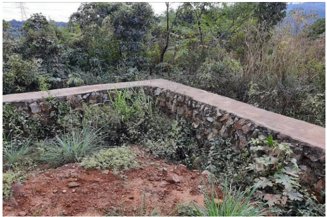
Retaining Wall at Tower AP-42A/0
