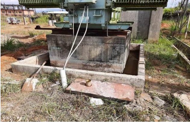
Oil Spill Containment Systems and Septic Tank at 33/11 kV Mynkre (new) S/S
