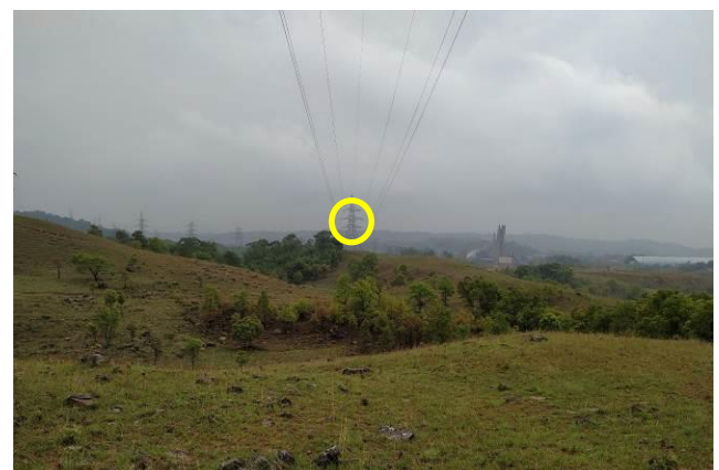
Tower on Hill Top to Minimize Tree Cutting
