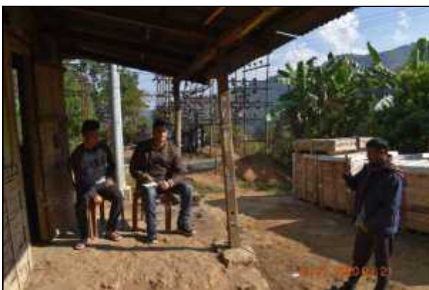
33/11 kV Substation at Changtongya
