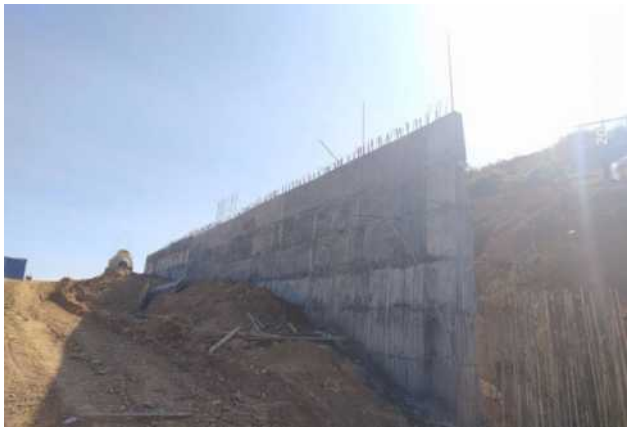
RCC Retaining Wall at 132/33kV New Secretariat Complex Sub-station
