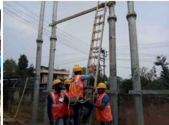
Training on Height Work
