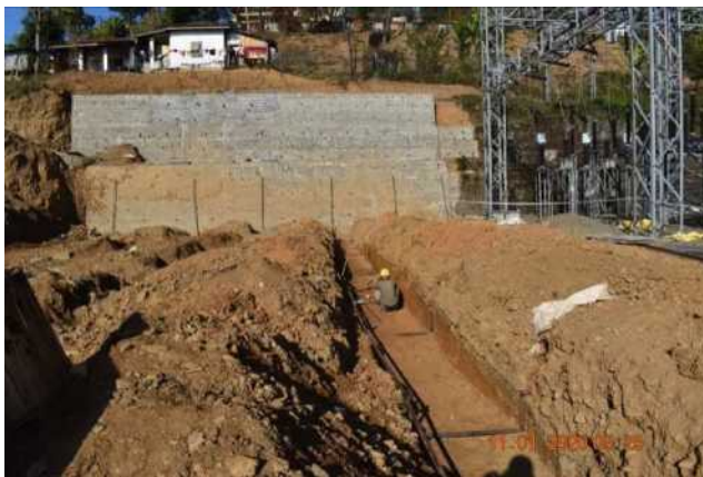
RRM Wall at 132/33 kV Mokokchung Sub-station
