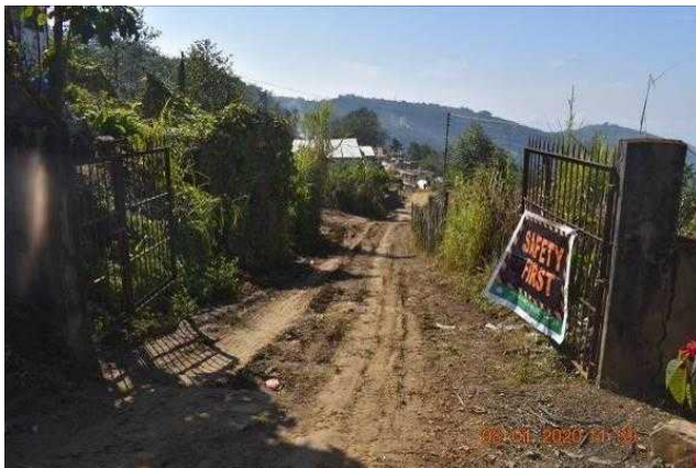
132/33 kV Wokha S/S Boundary Wall & Gate
