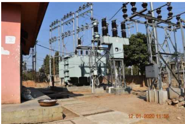
33/11 kV Substation at Industrial Estate (Augmentation)
