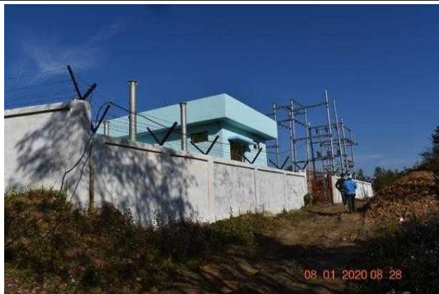
33/11 kV Chiephobozou S/S Boundary Wall
