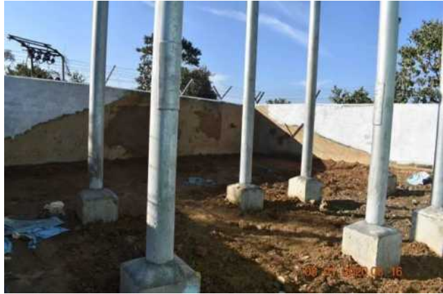
Refilling and leveling of excavated material at Chiephobozou Substation
