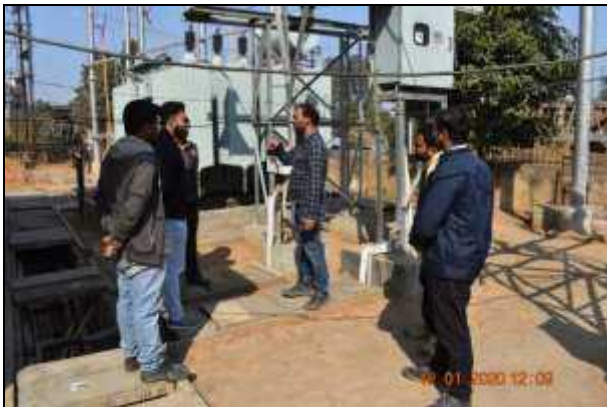
33/11 kV Substation at Industrial Estate
