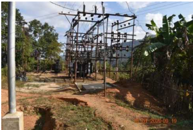
33/11 kV Substation at Changtongya (Augmentation)
