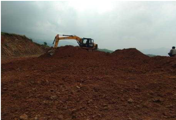
Cutting and leveling of excavated material at Zunheboto Substation
