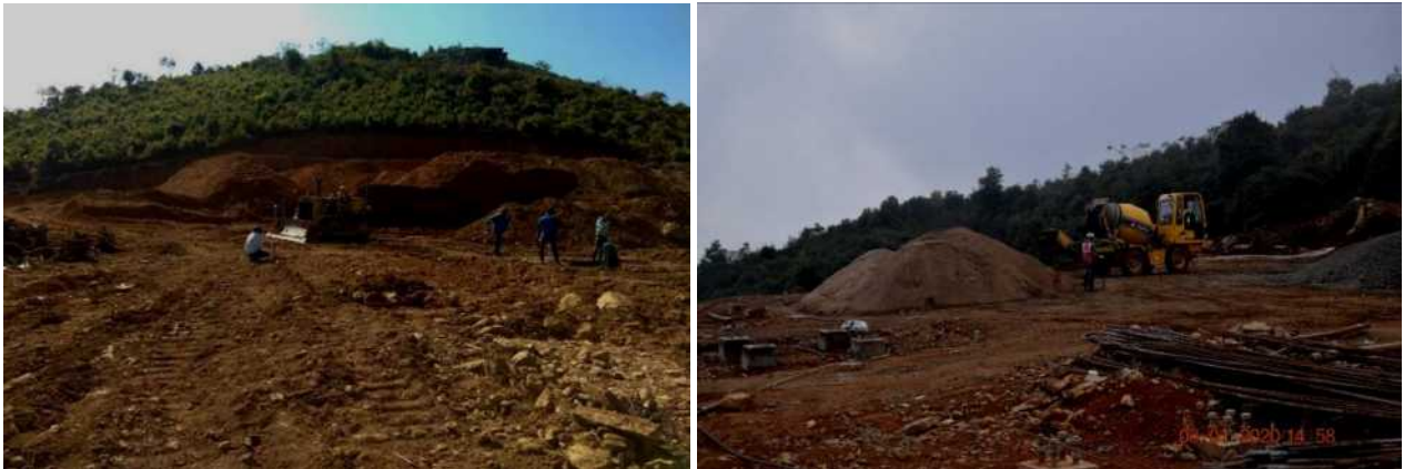
Earth cutting and Levelling at 132/33kV Secretariat Complex Kohima
