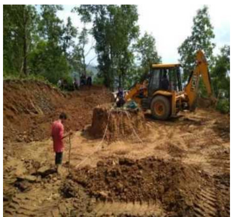
Refilling and leveling of excavated material after tower foundation and erection work
