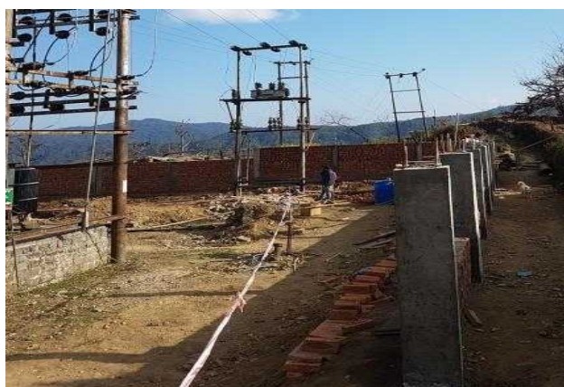
33/11 kV Pfutsero S/S Boundary Wall
