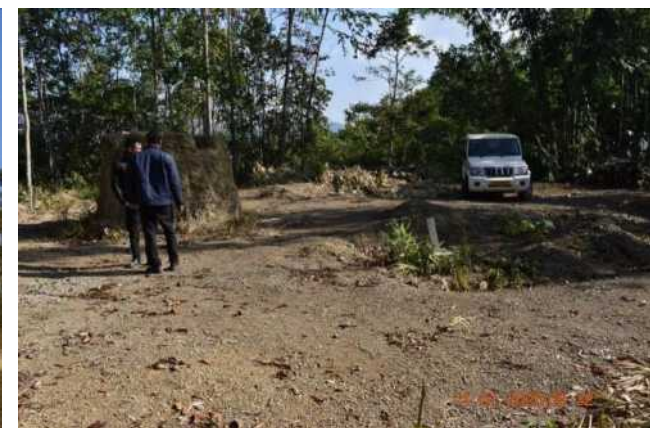
Tower Foundation at Mokokchung
