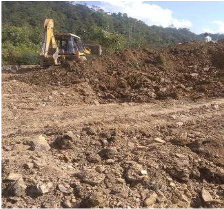
Refilling and leveling of excavated material at Chiephobozou Substation
