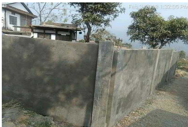
33/11 kV Lalmati (Zubza) S/S Boundary Wall
