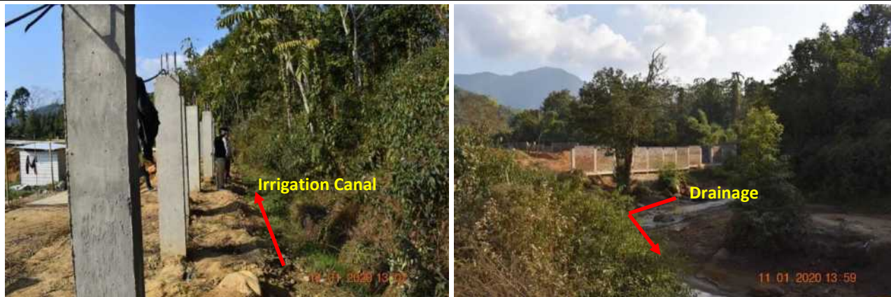
Protection/ Boundary Wall along the Irrigation Canal and Stream
