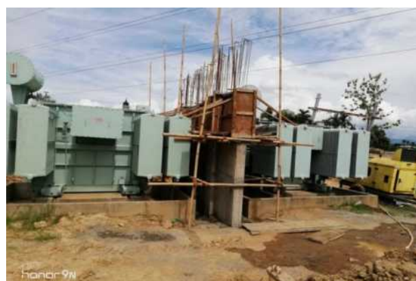
Fire Wall at Padampukhri
