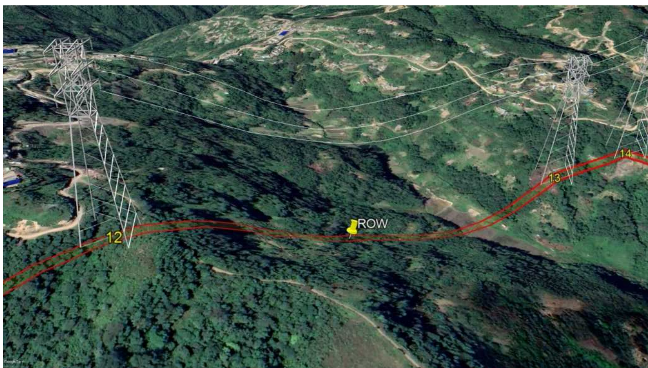
Figure 4.23: Increase in Length of Span Between Pole 12 and Pole 13
