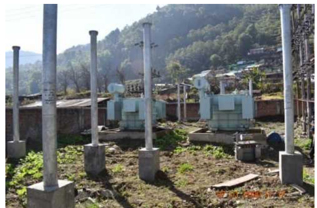
33/11 kV Substation at Pfutsero (New)
