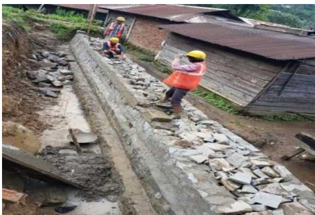
RRM Wall at 33/11 kV Pfutsero S/S
