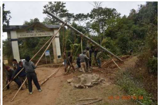
Pole erection work from Zunheboto South Point to Zunheboto
