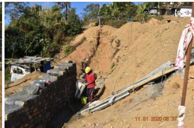
RRM Wall at 132/33 kV Mokokchung Sub-station
