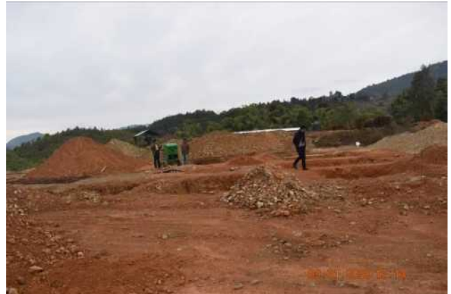
Cutting and leveling of excavated material at Zunheboto Substation
