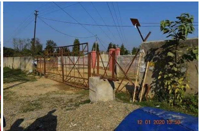
33/11 kV Padampukhri S/S B. Wall & Gate
