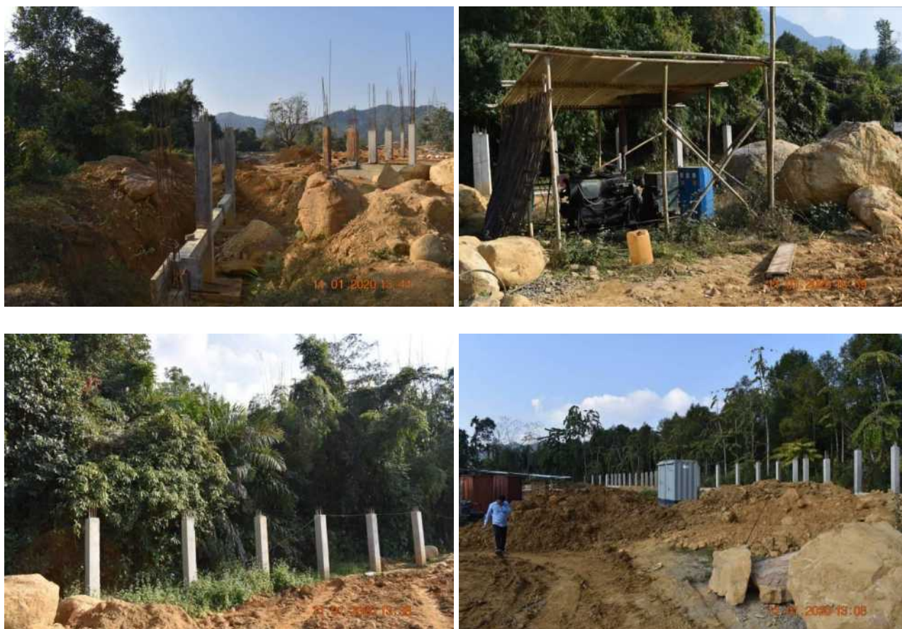
Unexpected excavation of boulders from 132/33 kV Lognak substation site
