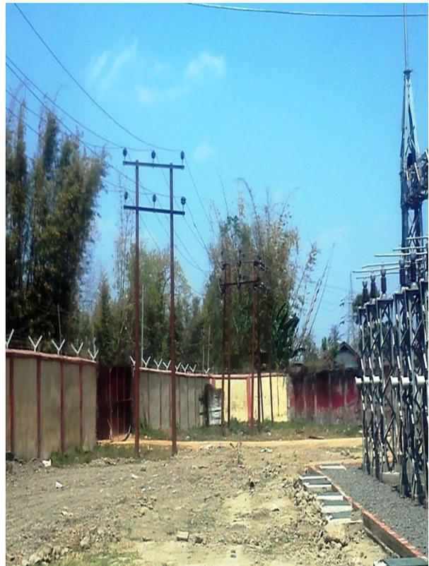
**33 kV (H Pole) line inside substation**
