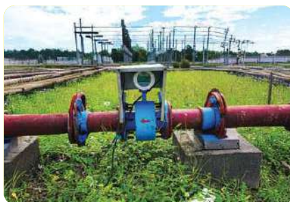
Digital Water Meter at Bishwanath Chariali S/s for accurate reporting of water consumption
