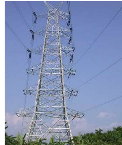
Narrow Corridor/Multi-circuit/Pole type towers minimising Right-of-Way
