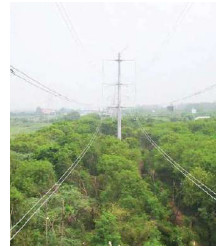
Narrow Corridor/Multi-circuit/Pole type towers minimising Right-of-Way
