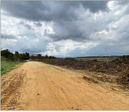
As part of the rejuvenation process, BDA has constructed diversion drains and temporary bund roads to separate the desilted portion of the lake and facilitate transportation of silt. DH PHOTO/ASRA MAVAD
