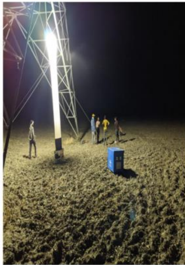
Restoration of 400KV Allahabad-Fatehpur#3 in night hours for broken Earth Wire.
