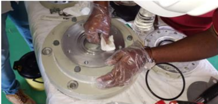
“ Departmental ” replacement of defective PRD in 400kV XIAN make “ GIS ” Bus reactor Isolator chamber at Tuticorin GIS with support from OEM through VC
