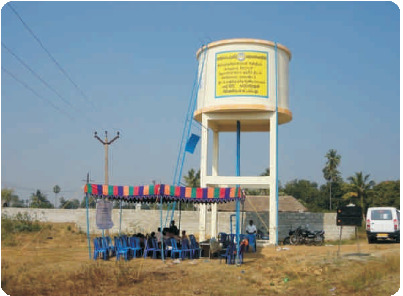
Overhead Water Tank
