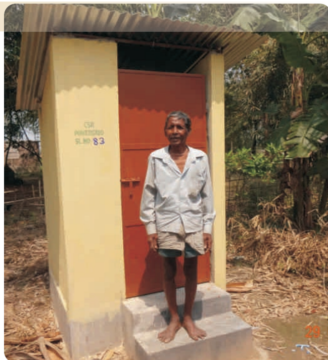
Low Cost Toilets at Simaluguri Village of Biswanath Chariali
