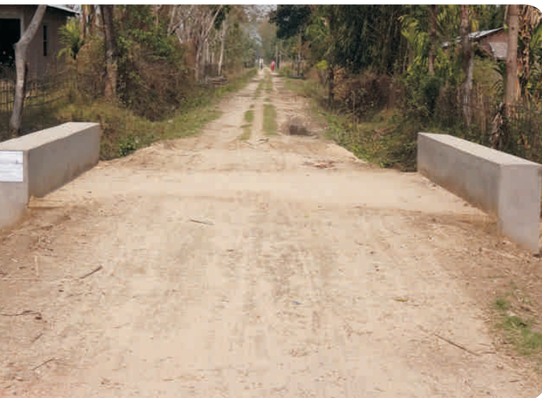
Culvert at Simaluguri Village of Biswanath Chariali
