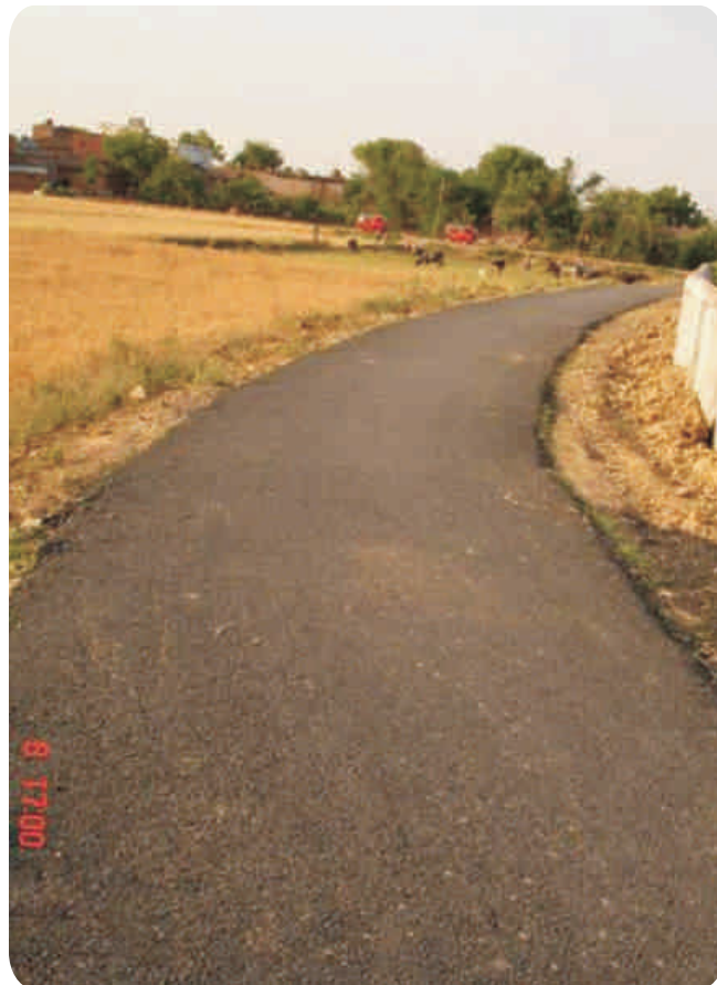
Repair and Maintenance of link road at Pusauli
