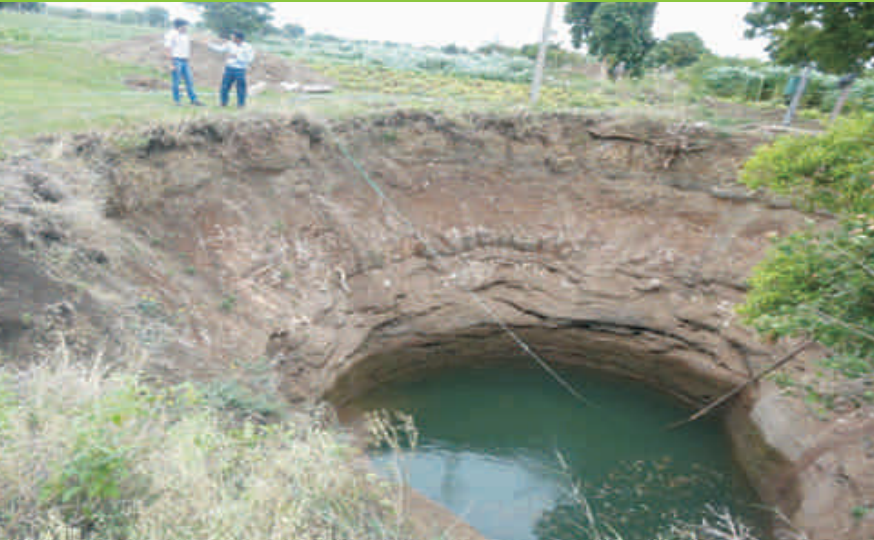
Dry well earlier: Now filled with water due to the watershed
