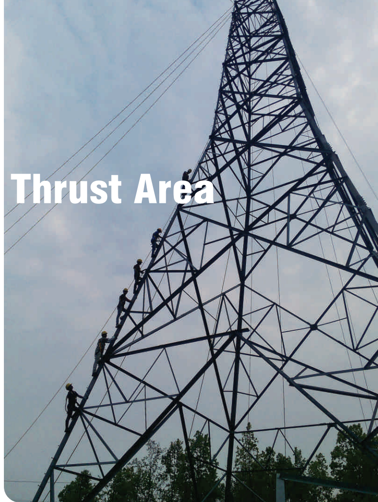
Capacity Building on Transmission Line Tower Erection and Stringing
