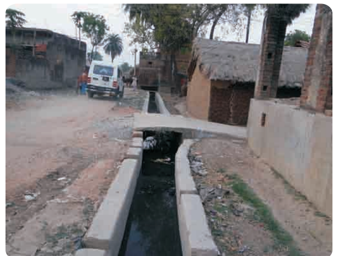
Renovation of drainage at Banka
