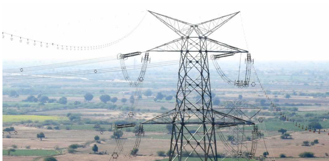
Bird diverters installed on POWERGRID line
