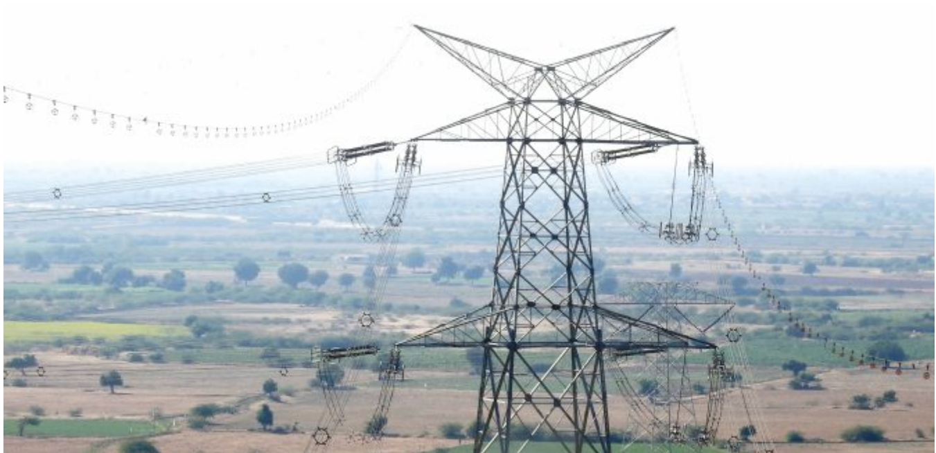
Bird diverters installed on POWERGRID line
