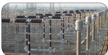
Indigenous Development of SF6 gas filled Current Transformer with BHEL
