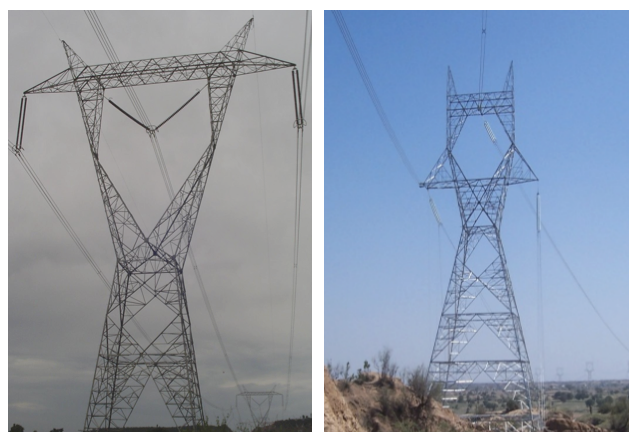
765 kV Horizontal Configuration - 85 mts. RoW
