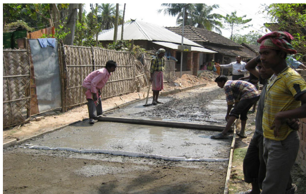
Construction of RCC road
