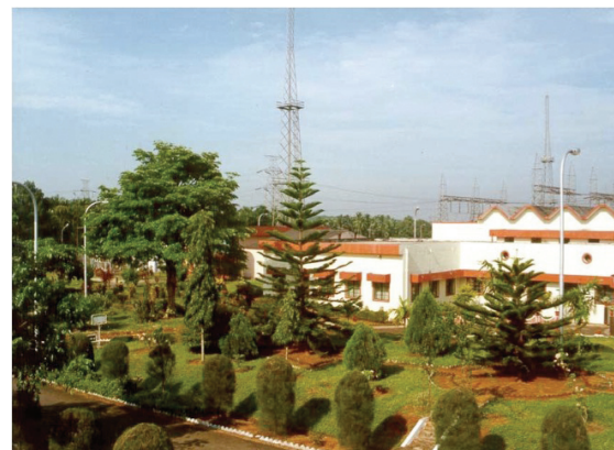
Top: Voluntary afforestation at Hyderabad substation.
