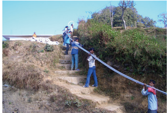
Transportation of conductors through head loads.
