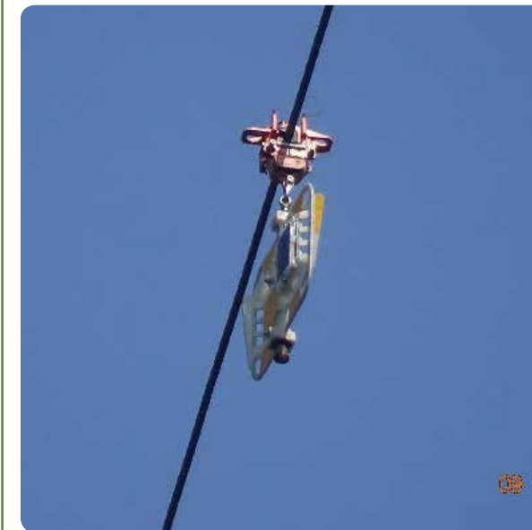
Bird Diverters installed in POWERGRID Transmission Lines for protection of Avifauna
