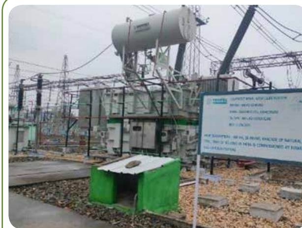
MAITHON SUBSTATION WITH REACTOR CONTAINING ESTER OIL
