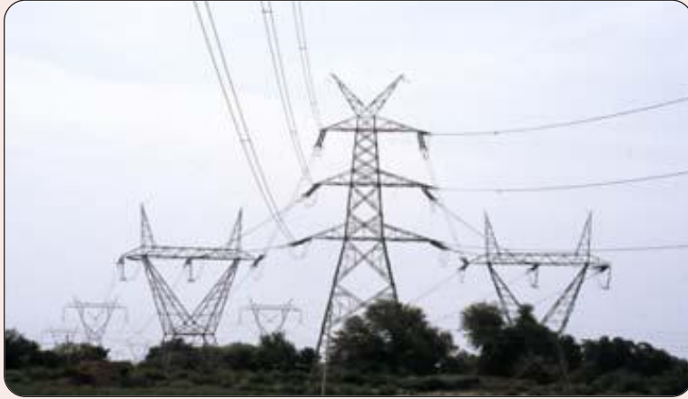
A view of transmission network
