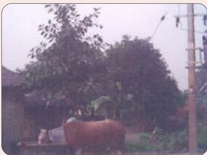
A view of Rural Electrification Network.
