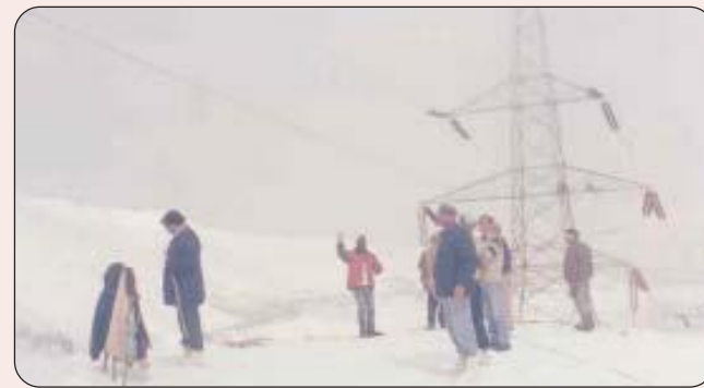
Men at work on 220 kv Pampore - Kishenpur line.
