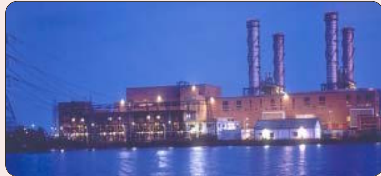
A night view of Gas Insulated Substation at Kayamkulam.
