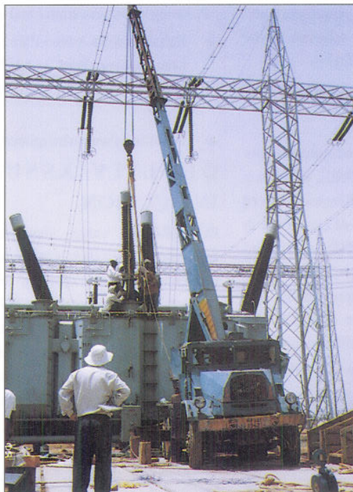
315 MVA-ICT-1 under erection in Bhiwadi Sub-station
