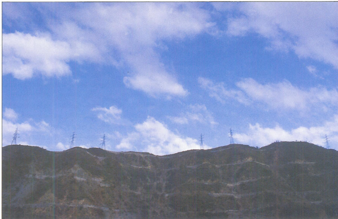
POWERGRID Towers - quest for higher excellence
