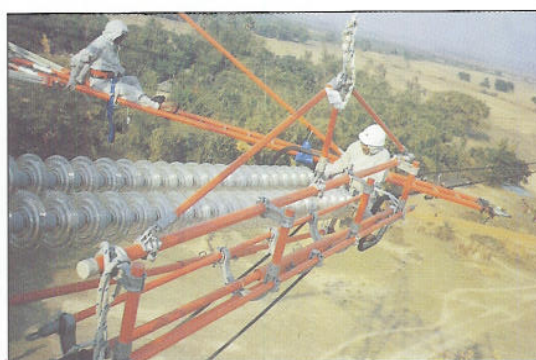
Hotline maintenance on 400 kV Farakka - Durgapur line in progress
