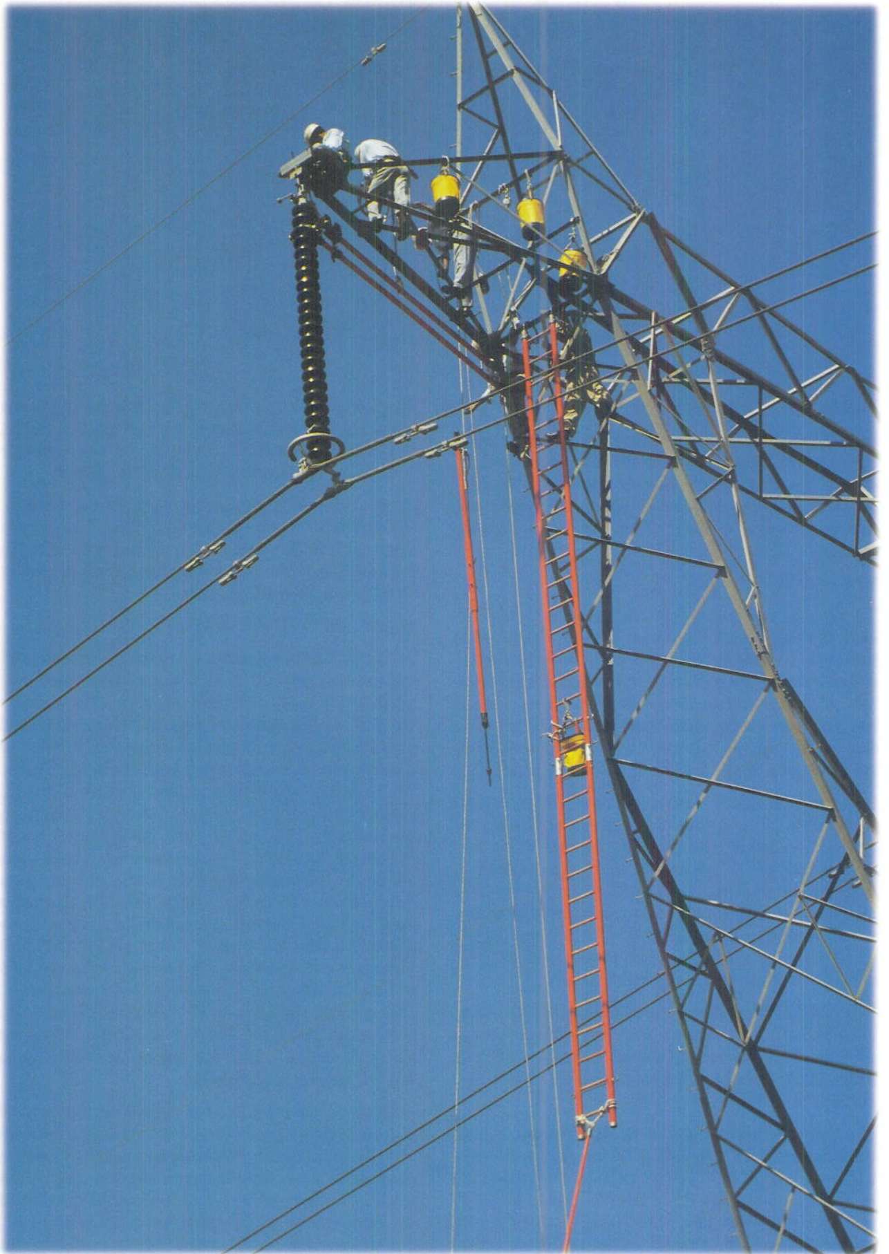
Hot line maintenance operation on 400 kV Indore-Asoj line
