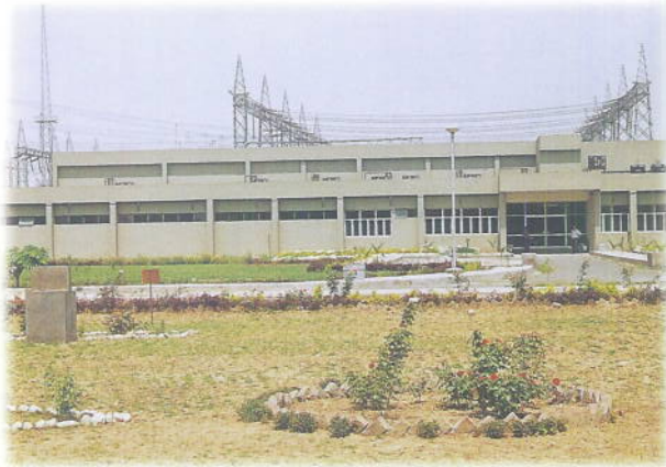
Control Room Building of 400/220 kV Abdullapur Sub-station
