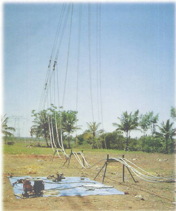
Stringing work \pm 500 kV HVDC Line in Talcher Transmission-System
