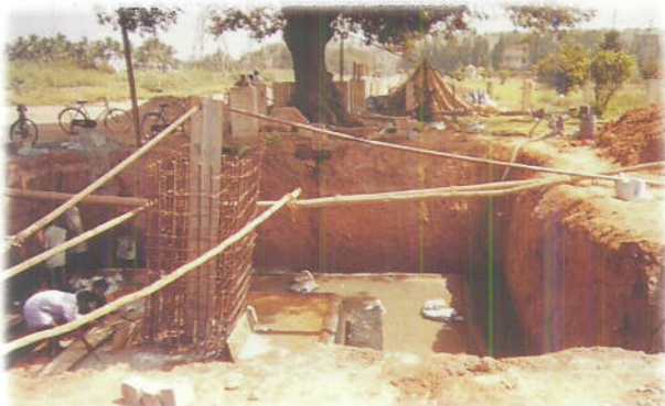
Microwave tower foundation work in progress at Neyveli
