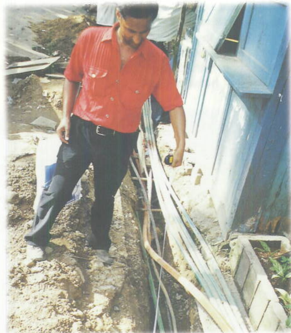
Underground installation of Optical Fibre cables
