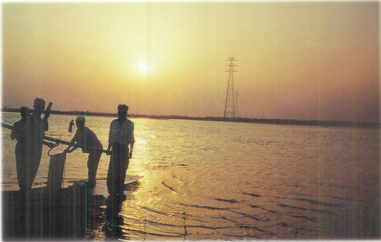
Sone River Crossing Tower of 400 kV D/C Biharshariff-Sarnath line
