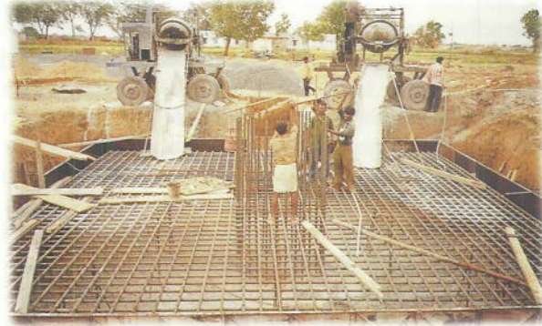
Pile Foundation work in progress in Talcher Trans. system
