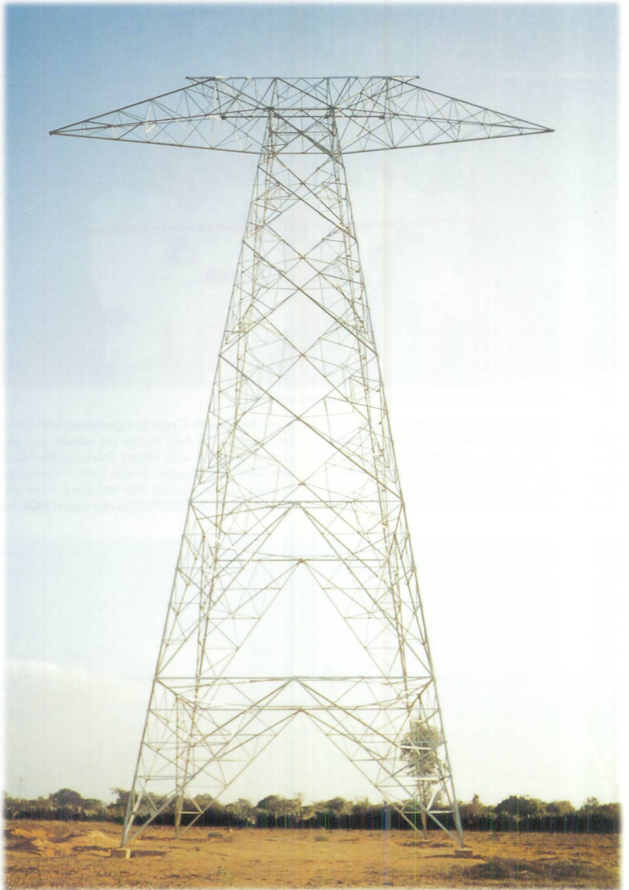
View of HVDC suspension tower
