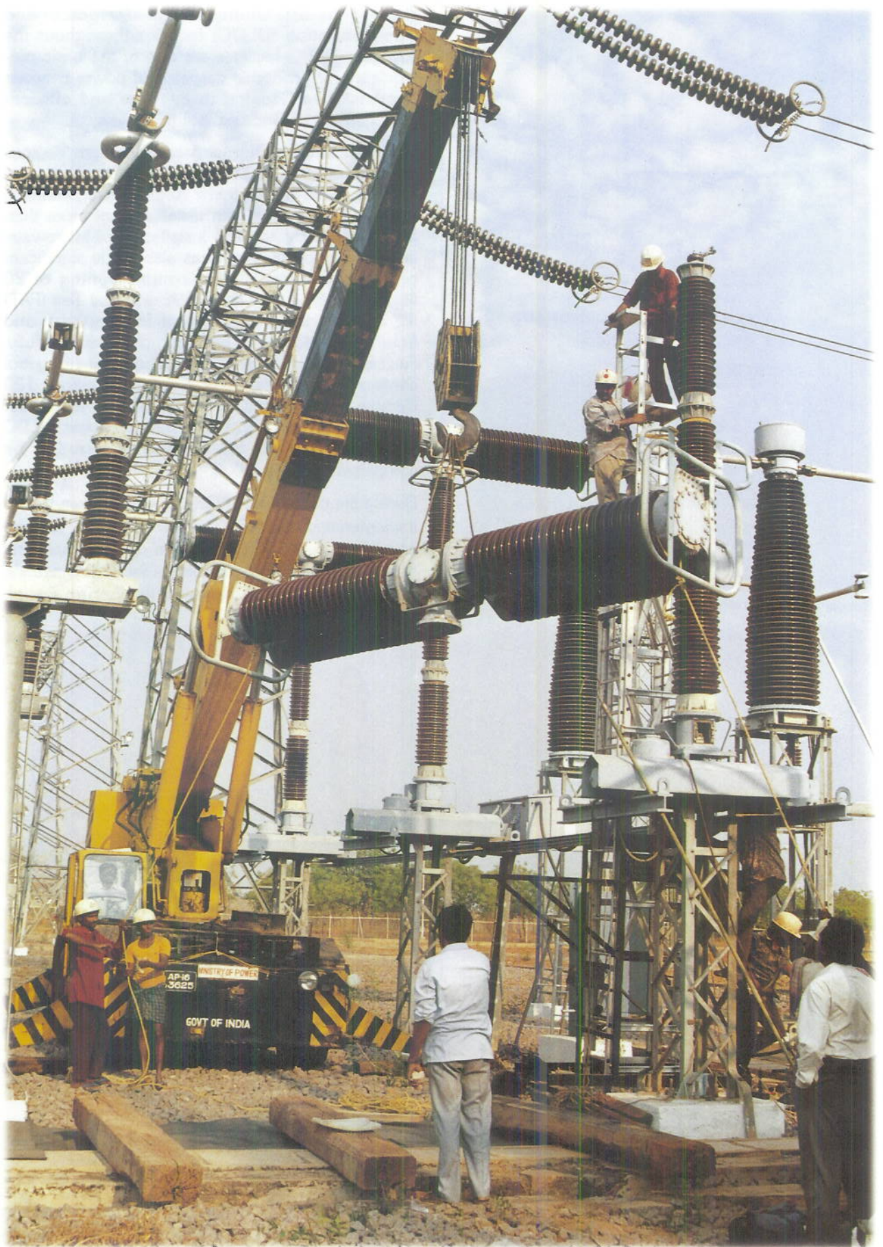
Circuit breaker overhauling in progress
