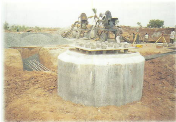
Pile Foundation work in progress in Talcher Transmission System
