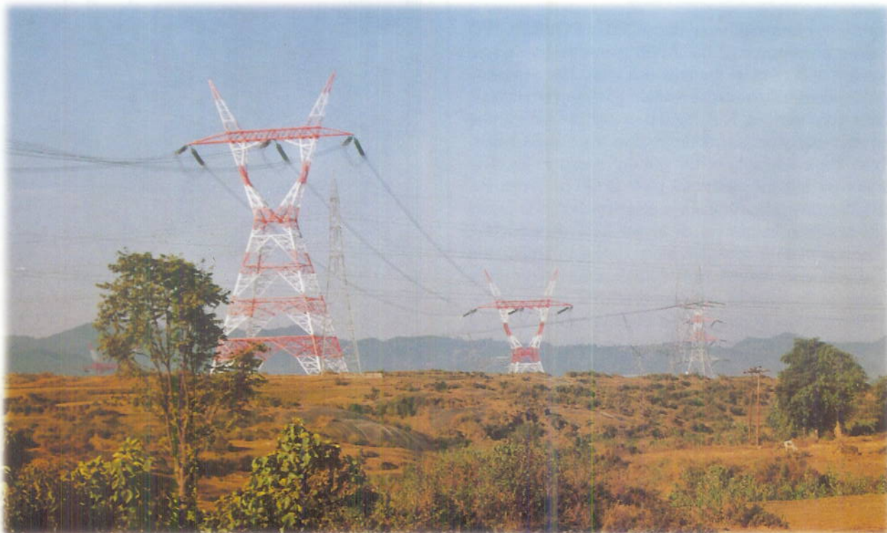
800 kV Kishenpur-Moga Transmission line
