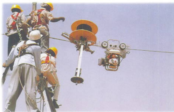
Wrap cable stringing work on Gooty - Bangalore 400 kV line
