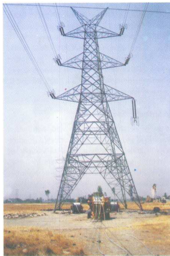
Stringing of conductor in Nalagarh-Hissar 400 kV D/C line in progress
