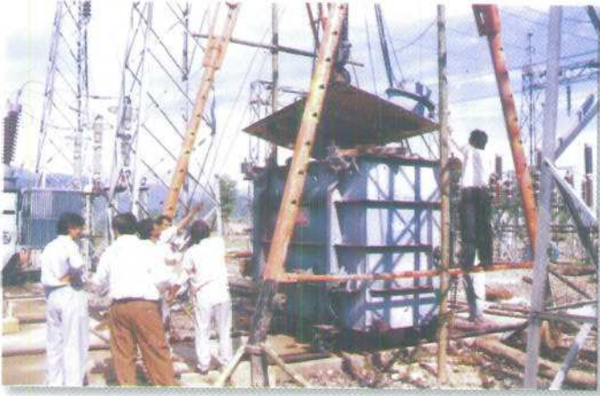
In-house repair work of 132/33 KV, 10 MVA Auto Transformer at Nirjuli Sub-station
