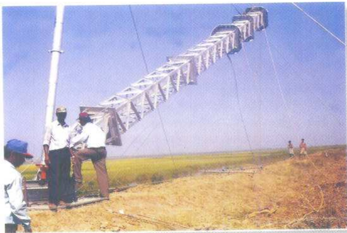
ERS being installed to restore power supply in Orissa
