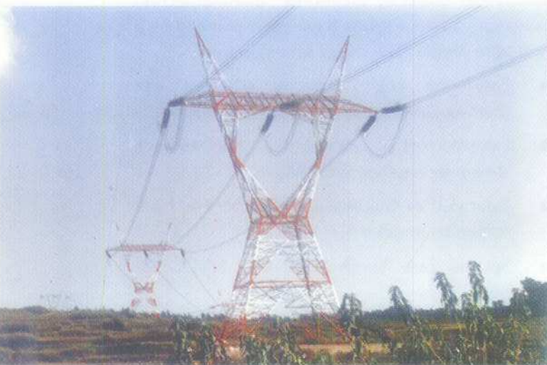
View of 800KV S/C Kishenpur-Moga line
