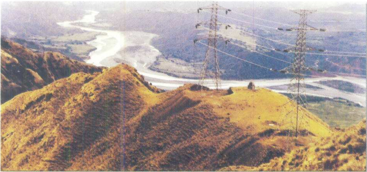
Aerial view of 400 kV D/C Chamera-Moga line.
