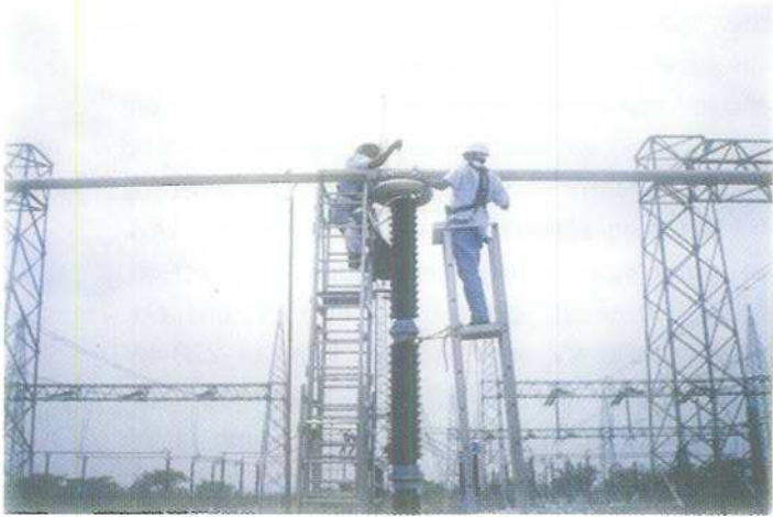
Bus Bar Maintenance at Khammam S/S
