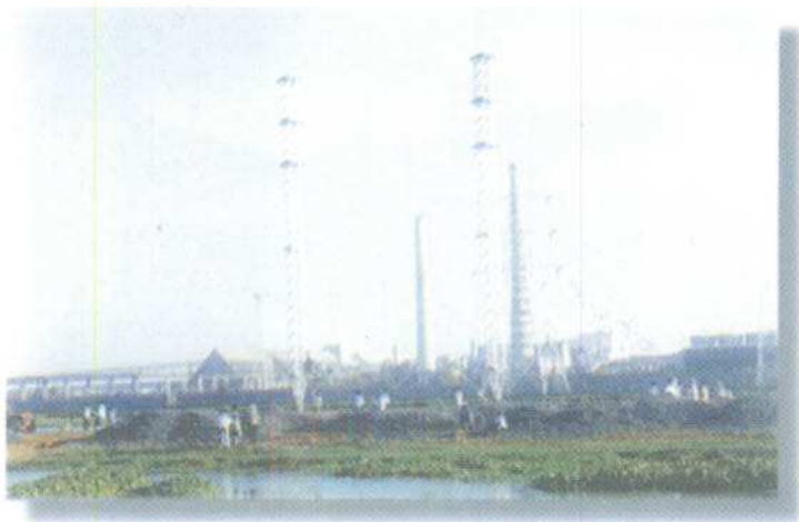
ERS on 132 kV Paradeep-Paradeep Phosphate line
