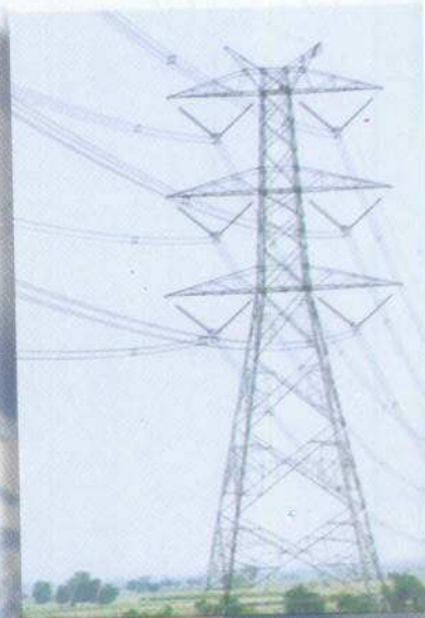
OPGW Cabling completed
