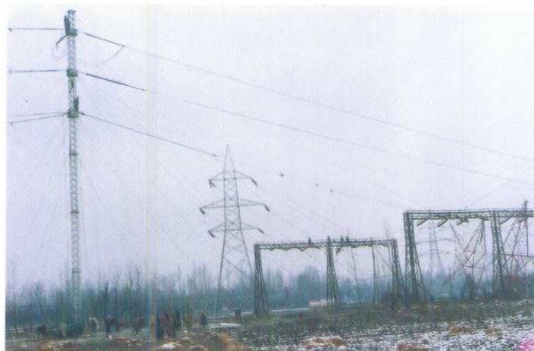
Restored through ERS on 25.1.2000.
