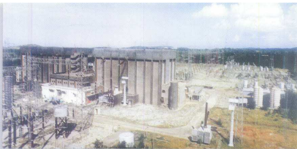
View of HVDC Rihand Project
