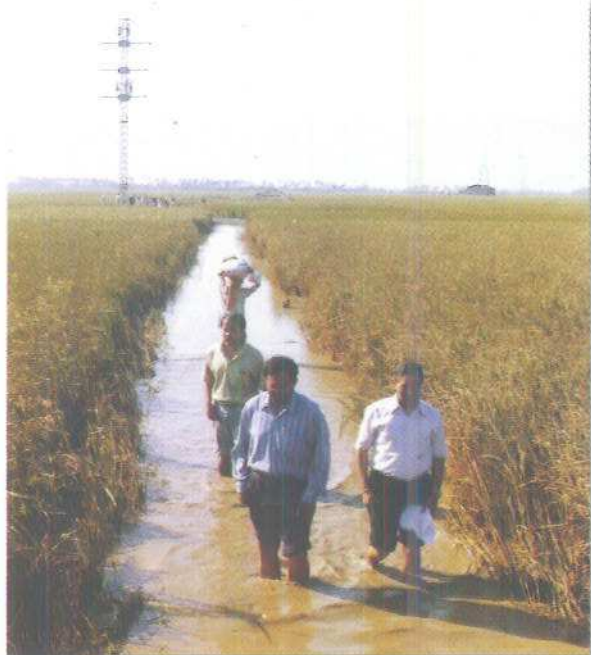
POWERGRID men at work to restore Kendrapara-Paradeep line after Orissa cyclone
