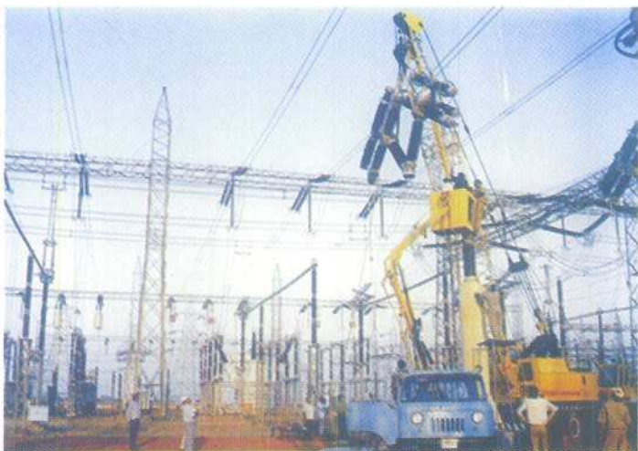
A view of Breaker Over-hauling in 400 kV Bhilai Sub-station
