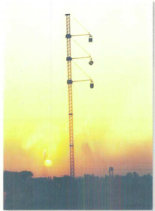
View of Emergency Restroration System during sunset
