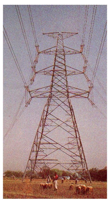
Quietly co-existing-Two circuits of a 400 kv Transmission Lines pass over the country side.
