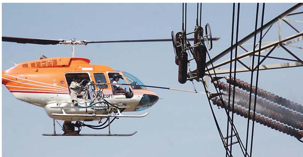
was carried out by POWERGRID. This highly sophisticated technique was implemented by deploying helicopter on 12 transmission lines in heavy polluted stretches for a period of five months (Nov'08 to March'09). The results are encouraging as the trippings reduced on above mentioned transmission lines.
