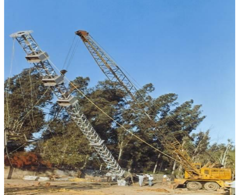
Emergency Restoration System (ERS)
