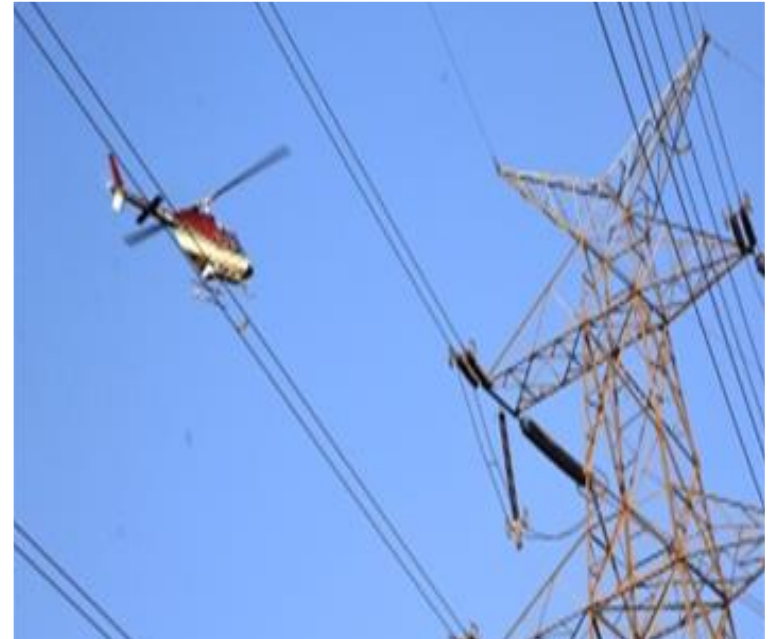
Aerial Patrolling using Helicopters
