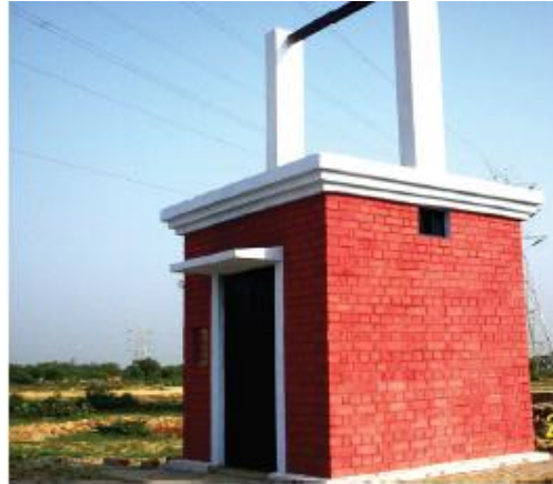
Tubewell in Lucknow Under CD Works
