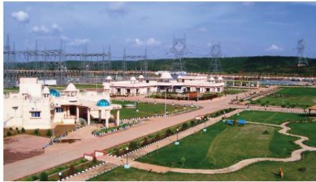
Gwalior S/S After Construction
