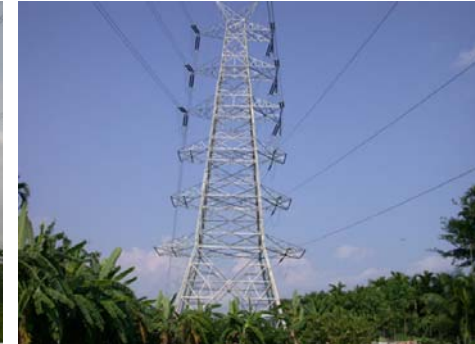
Multi Circuit Tower in Forest
