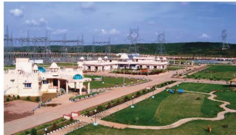
Gwalior S/S After Construction
