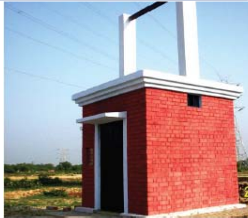
Tubewell in Lucknow Under CD Works
