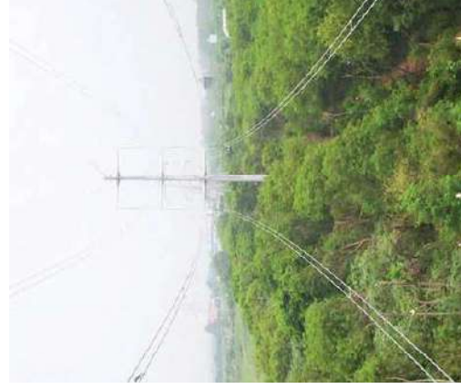
Narrow Corridor/Multi-circuit/Pole type towers minimising Right-of-Way
