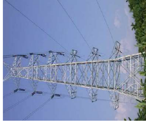
Narrow Corridor/Multi-circuit/Pole type towers minimising Right-of-Way
