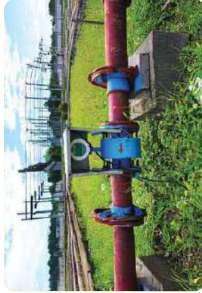
Digital Water Meter at Bishwanath Chariali S/s for accurate reporting of water consumption
